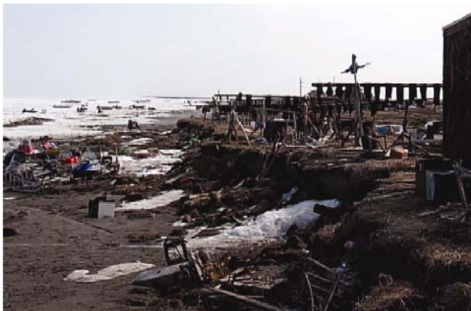
Sea erosion and permafrost melting in Shishmaref, Alaska
